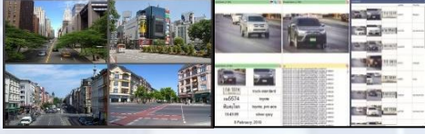
Monitor CCTV and License Plate
