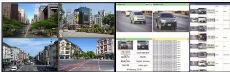
Monitor CCTV and License Plate
